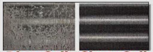
Dirty Coil Clean Coil
